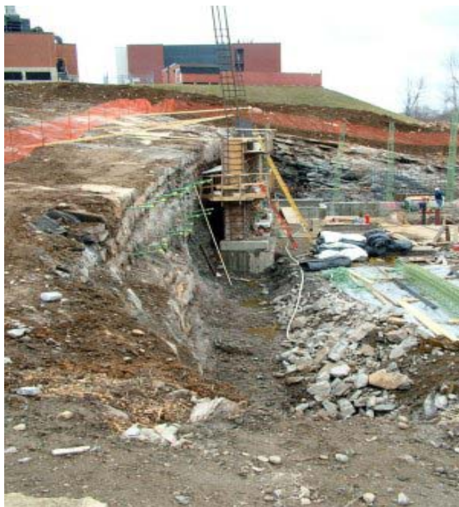
CONSTRUCTION BEGINS FOR NEW ESCAPE TOWER
